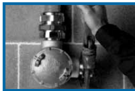
5. Install hub on enclosure
