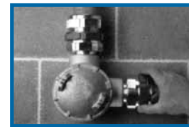
6. Insert cable and tighten red union
