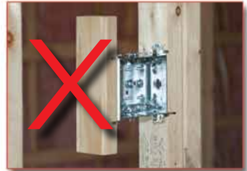
This installation does NOT COMPLY with C.E.C. 12-3010 (3).
